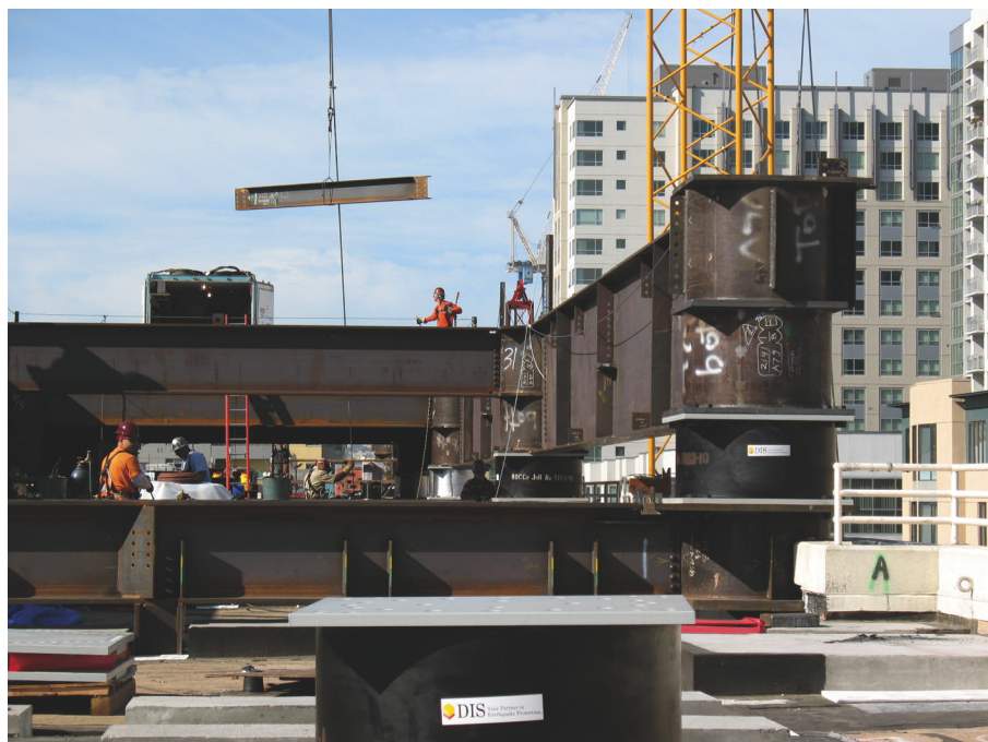
The seismic isolator can be seen in between the two structural steel grids.
